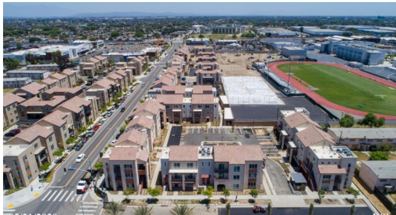
Figure B1: Areas 1A, B, and C completed with the updated extension of Century Blvd.
