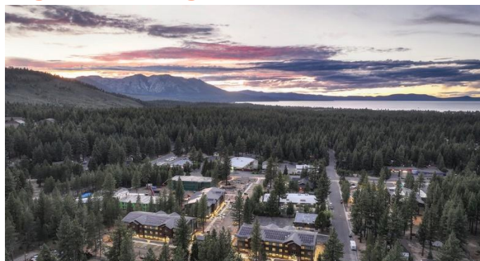
Figure C1: Sugar Pine Village Aerial view with Phase I and II complete.
